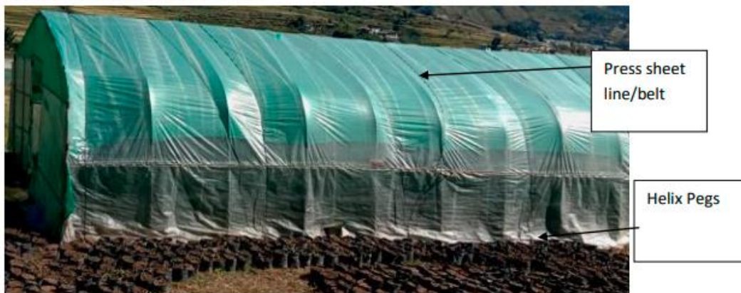
Figure 1c. Outer view of poly house
