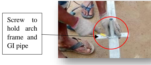
Figure 2. Fixing of screw on the arch frame and GI pipe
